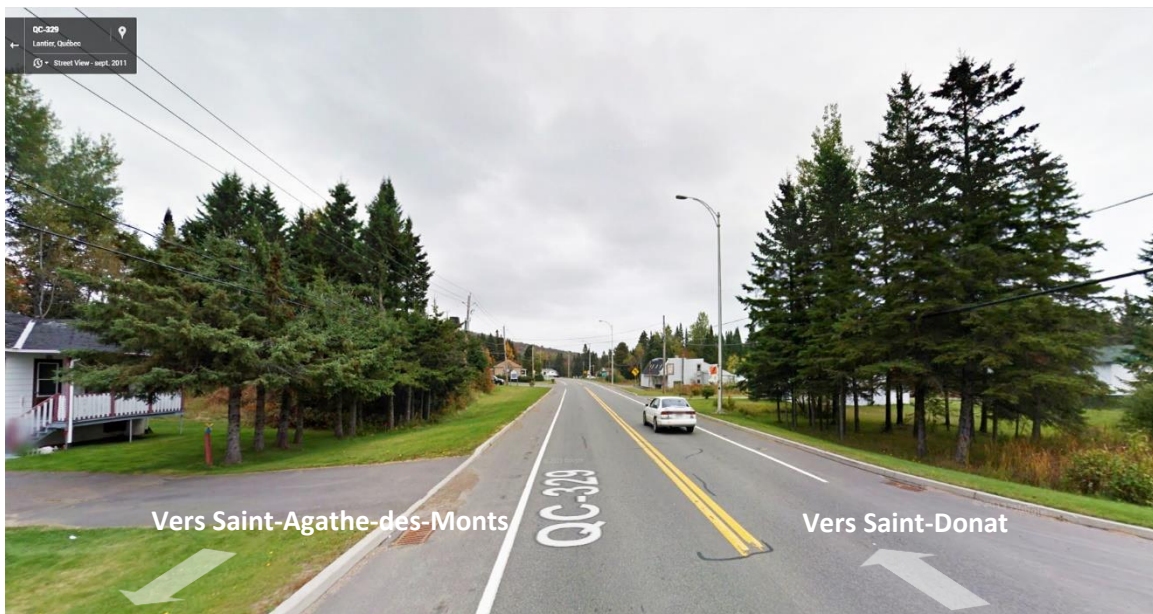
Source: Google Street view – Google Maps
